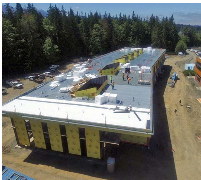
Aerial View of Allied Health and Early Childhood Development Center under construction
